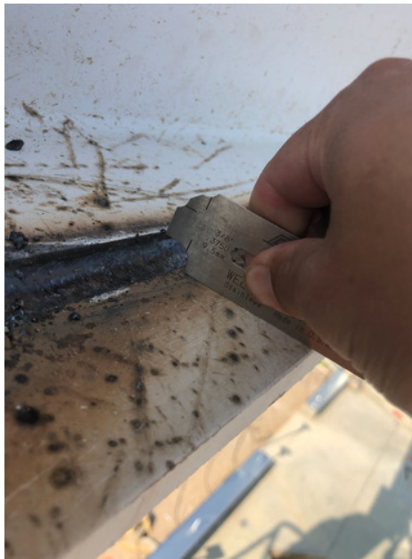
Fig. 4: Column to beam fillet weld
