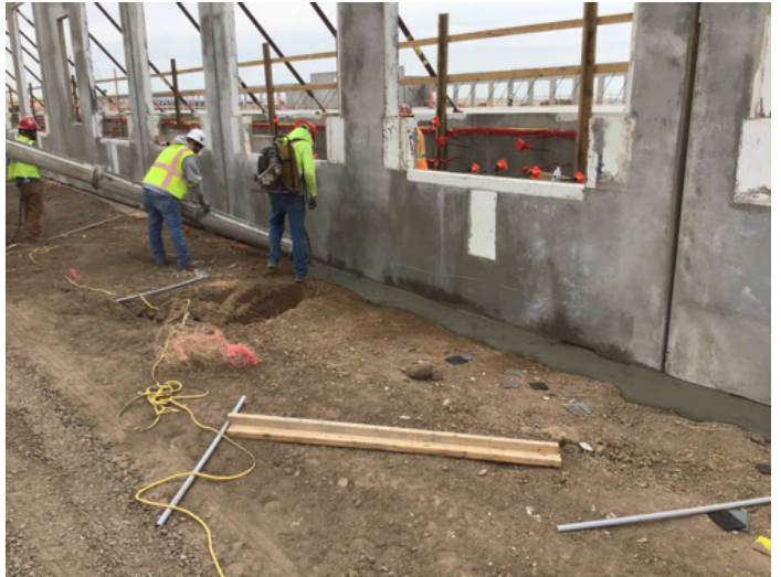
Fig. 4: Outside of wall grout
