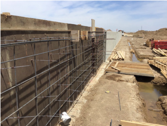
Fig. 3: Rebar being placed
