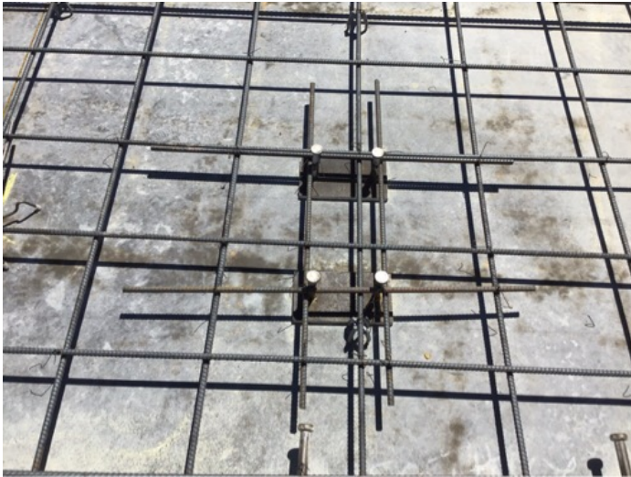
Fig. 1: Canopy inbed plates
