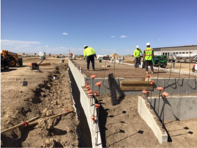
Fig. 1: Guard Shack foundation prep
