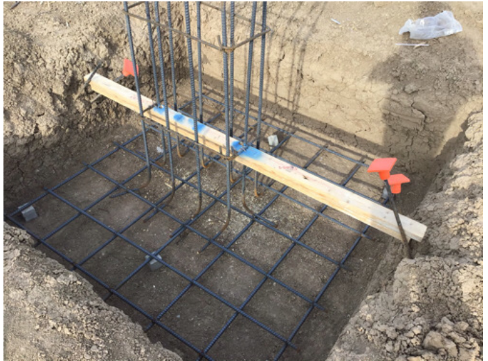
Fig. 6: Footing for guard shack
