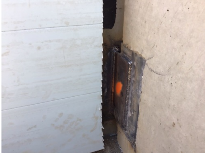
Fig. 4: 4X8 plate weld to plinth corner North office area
