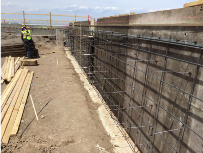
Fig. 1: Rebar placed
