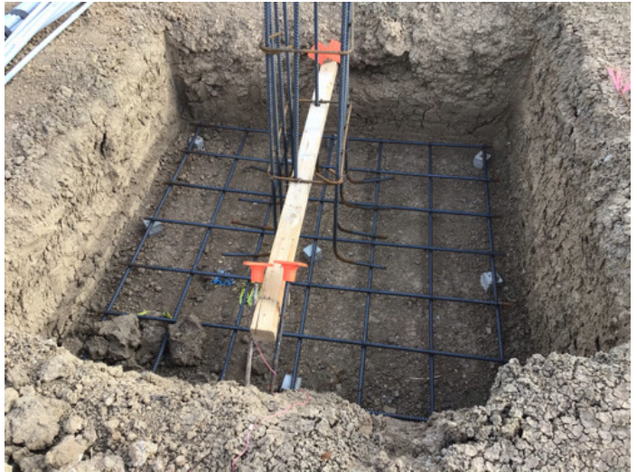
Fig. 8: Footing for guard shack
