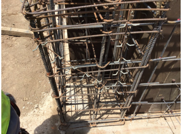
Fig. 2: Rebar being placed
