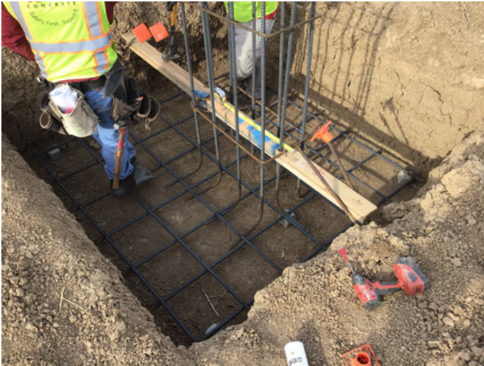
Fig. 5: Footing for guard shack
