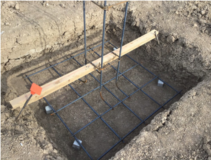
Fig. 7: Footing for guard shack
