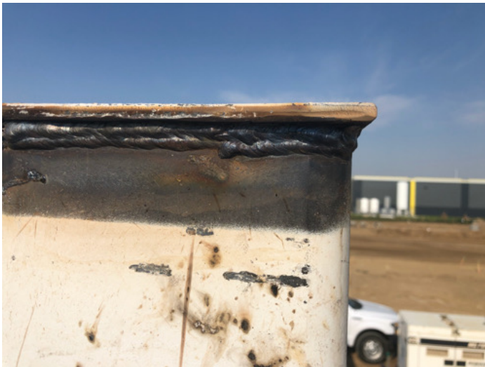
Fig. 3: Top of column cap weld
