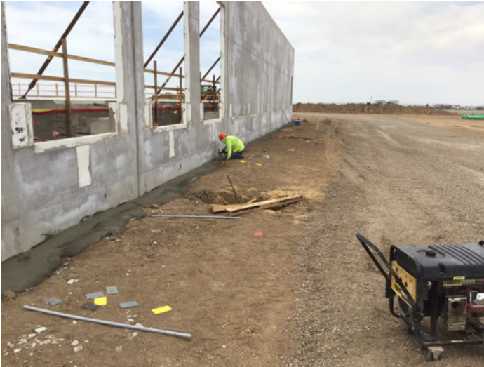
Fig. 3: Outside of wall grout
